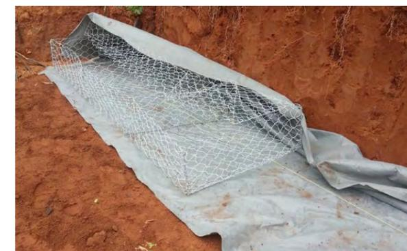
Figure 21 showing installation of gabion baskets
