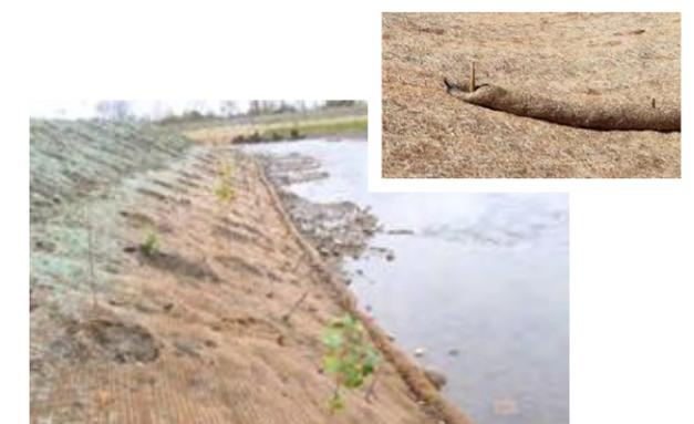
Figure 19: A photo showing the initial sloping and revegetation phase
