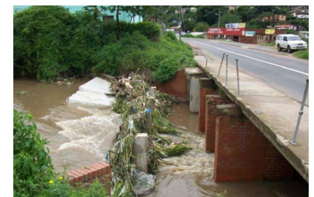
Figure 16 and 17 showing examples of debris walls that have been constructed upstream of culverts/bridges
