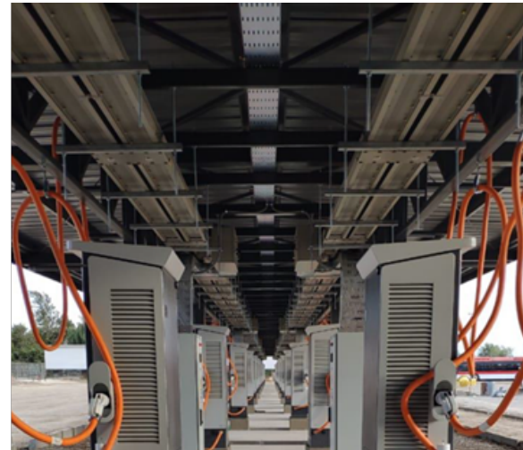
Figure 8. Example of how charging infrastructure can be built into the roof to lessen space requirements.
